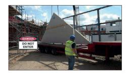
7. The crane will then take up the slack of the lift. On instruction from the site responsible person the driver will release the transport straps on the side being unloaded.
