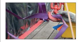
9. The crane will then lift the panel from the bed of the trailer. Given the weight and shape of panel it is essential that the danger area in front of the panel is kept clear of all personnel. **NEVER** stand in the danger area where the panel could potentially fall or swing. Do not allow any others to enter the danger area.
