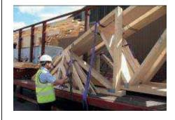
**3**. The manufacturer will supply truss packs secured to the trailer with 8mm blue rope. You should familiarise yourself with which rope attaches which pack to the centre bars.
