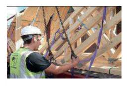
2. Trusses will arrive pre-slung with appropriate 7:1 lifting slings. These slings will be reachable from ground level and should be deemed as single use
