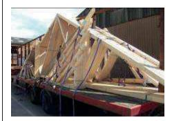
5. Once the order of unloading is agreed between the slinger and driver, the slinger will attach the purple lifting slings to the crane hooks
